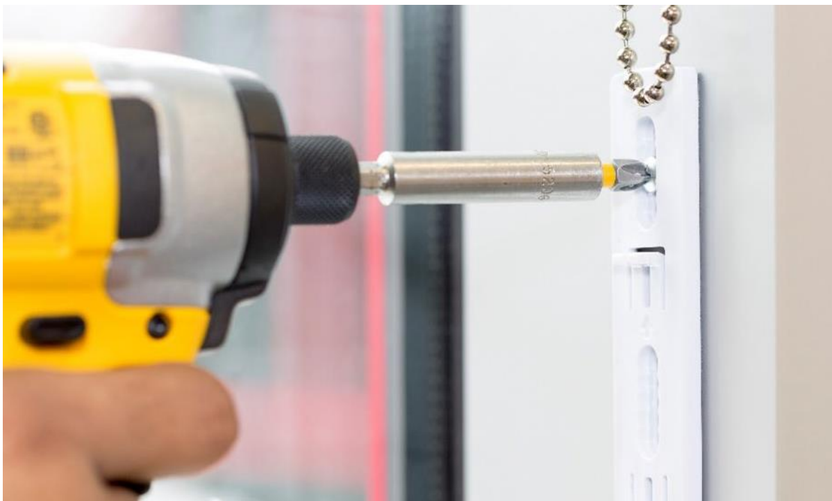
Picture 16-Fixing Mounting plate
